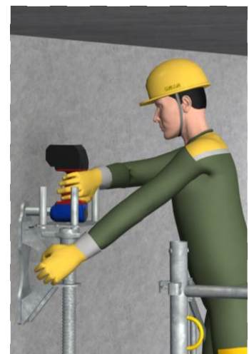
2.5T Wall bracket removal
