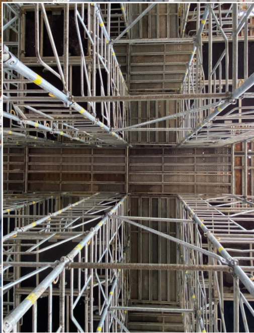
Touréchaf falsework for the construction of the primary settling unit of the Achères water treatment plant.
