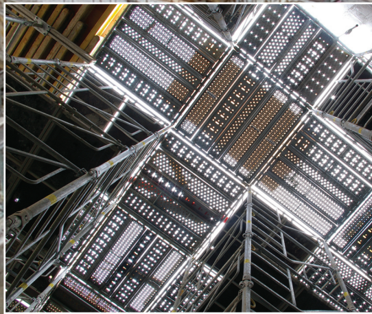
Touréchaf falsework with decking between towers for girder formwork, Delessert passage in Paris.
