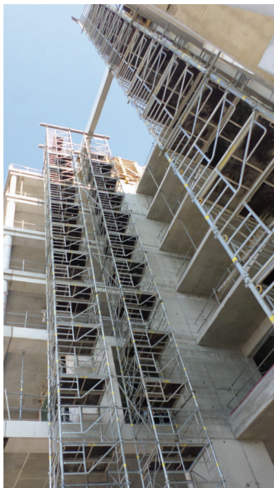
High-height Touréchaf falsework for the erection of the head office of Caisse d'Épargne in Bordeaux.
