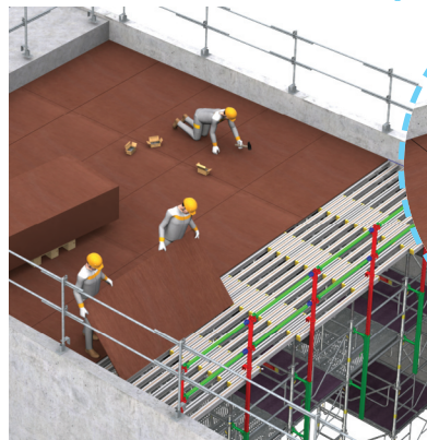
> 8 - Lay the plywood. The MP3 beams as secondary beams make the operator's displacement safe.
