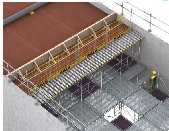
> 4 - Install the decking between the first and second part of the falsework.
