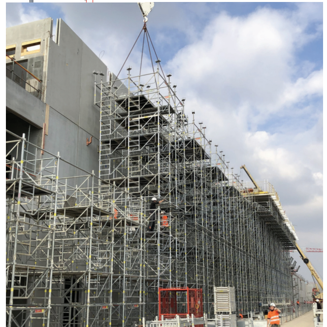
Stacking Touréchaf for the future operation centre of lines 16 and 17 of the Grand Paris Express in Aulnay-sous-Bois.
