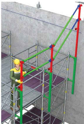
> 4 - Continue the assembly in the next mesh by installing an upright and two ledgers.
