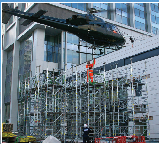
A Touréchaf being lifted by helicopter using the lifting rings to the top of a 100 m high tower.
