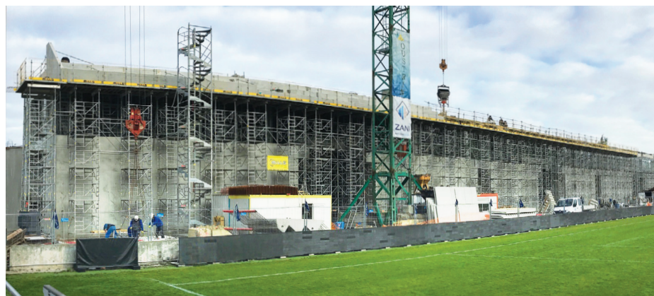
Touréchaf falsework tower for the construction of the Armandie grandstands in Agen.
