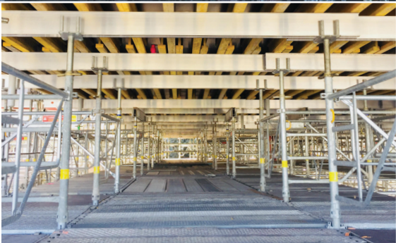
Decking at the top of towers for fitting and removing formwork in safety.
