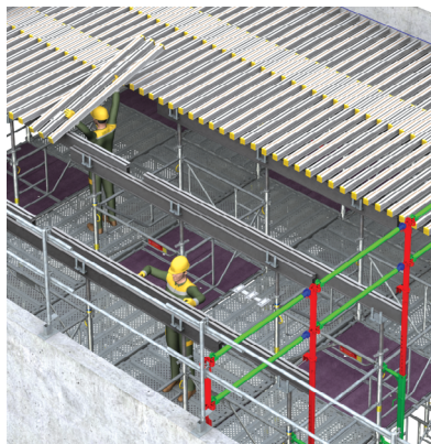
> 7 - Install the beams.
