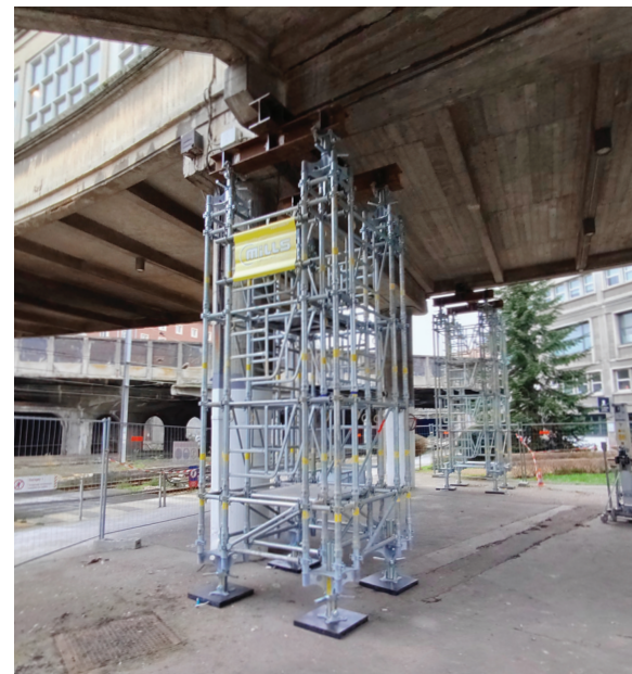
The access footbridge to the platforms of the SNCF railway station in Amiens is back propped.
