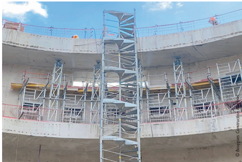
Touréchaf Pylon for a structure in Vitry-sur-Seine.
