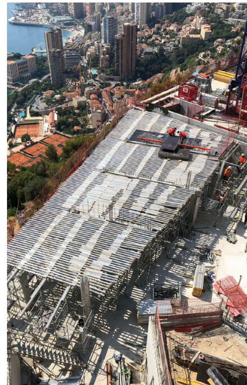
Touréchaf falsework equipped with MP3 formwork aluminium beams for the construction of the Vista Palace - La Cigale Hotel at Roquebrune-Cap-Martin near Monaco.
