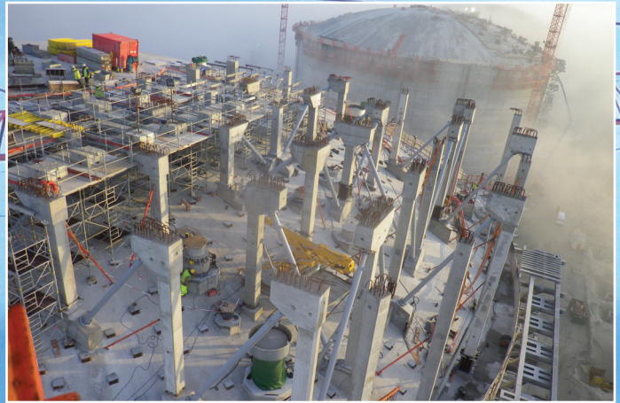
Touréchaf falsework for carrying out girders at 50 m in height on domes of the 3 tanks of the methane terminal (LNG) on the seafront in Dunkerque.
